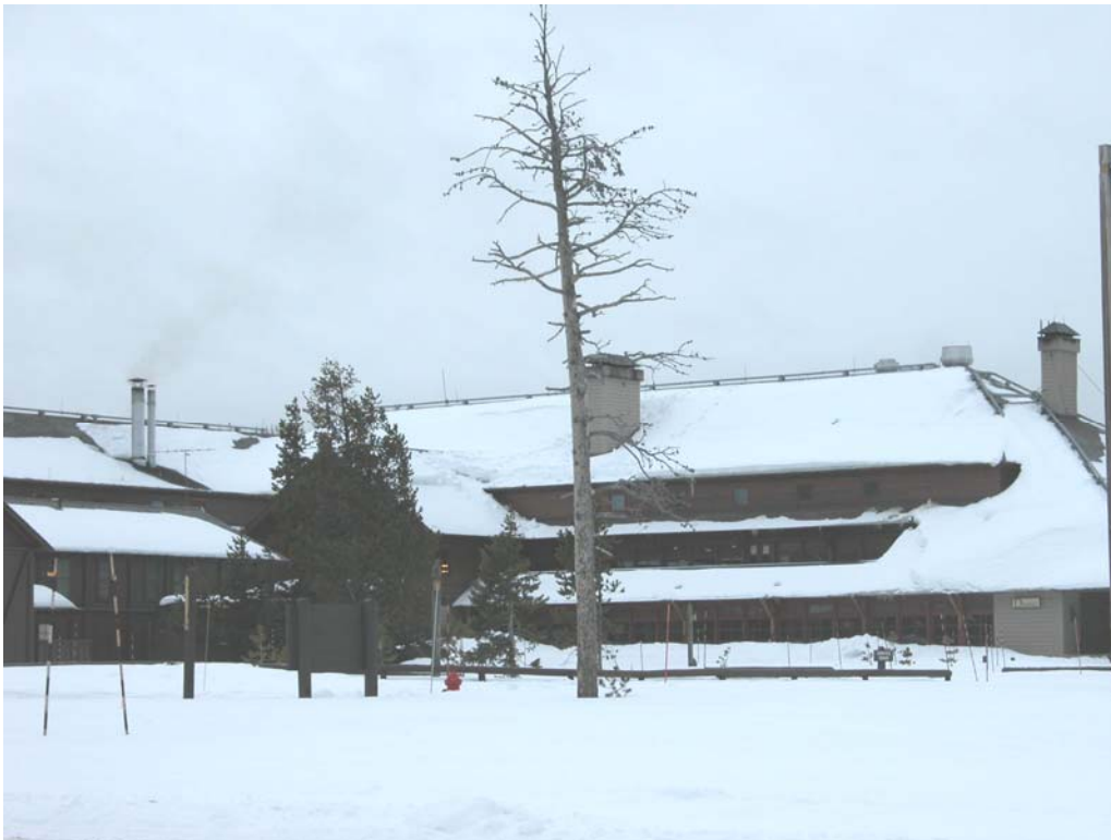
View of Snow Lodge to the south of the monitoring shelter. Smoke can be seen raising from the boiler room. The two large stacks are from the gas-fueled public area fireplaces which do not produce visible plumes. During the evening, smoke can be seen coming from the kitchen vents that are on the far side of the roof, right side.
